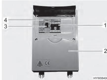
Fig. 102 230 V fuse box with safety cut-out and FI-switch
