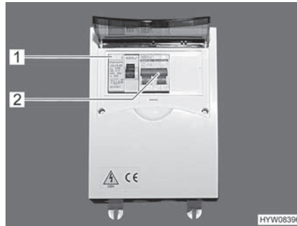
Fig. 119 230 V fuse box with safety cut-out and FI-switch
