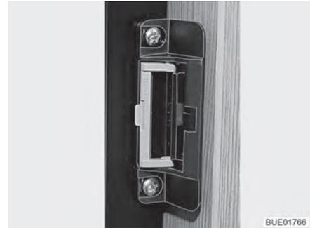
Fig. 102 Locking device in ventilation position
