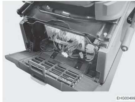
Fig. 76 Transformer/rectifier position (Stellantis)
